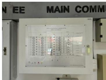
Fire Alarm Control Panel
